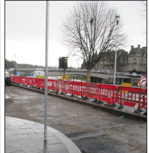
Road reconstruction work on Bank Street
